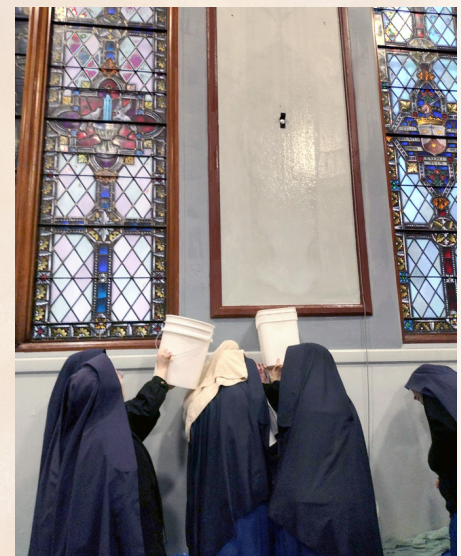
Sisters rushed to help when sub-zero temperatures caused a pipe to freeze above the ceiling of Mount St. Michael's chapel, resulting in a waterfall.
