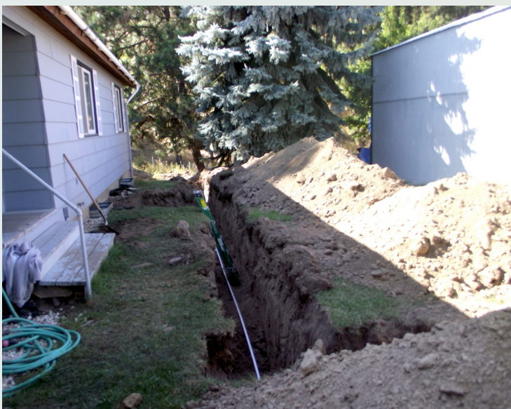
Huge ditches were dug in the grounds around the Novitiate this fall as water and electrical lines were placed so that the Sisters can have farm animals.
