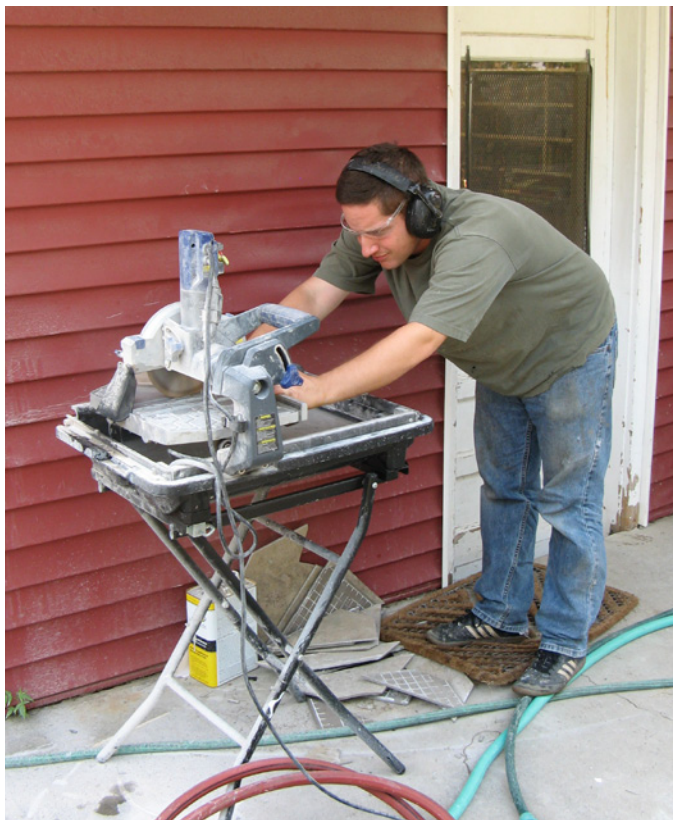
Frater Philip cuts tile to proper size
